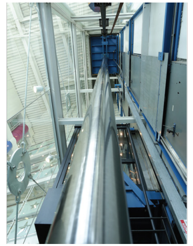
S-9 Hidrolik L Karkas L Frame For Hydraulic Lift
